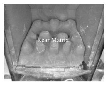
Locate the LEFT HAND and RIGHT HAND FRONT PEBBLES as shown so that they sit on the front rail and lean back against the BASE MATRIX. Note it is most important that they are located in their correct positions. They are marked on the rear "L" for LEFT HAND FRONT PEBBLE and "R" for RIGHT HAND FRONT PEBBLE.
